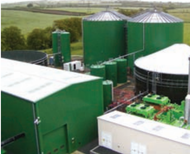
Holsworthy Biogas Plant
